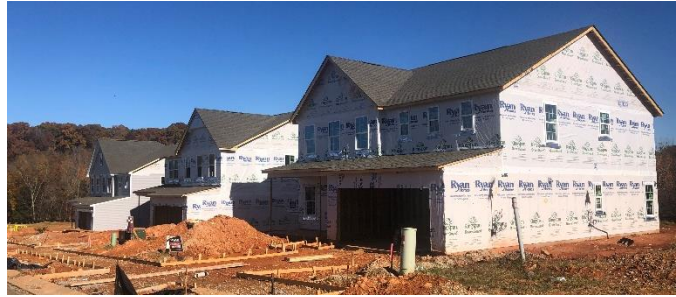
New-home construction in a Concord neighborhood
